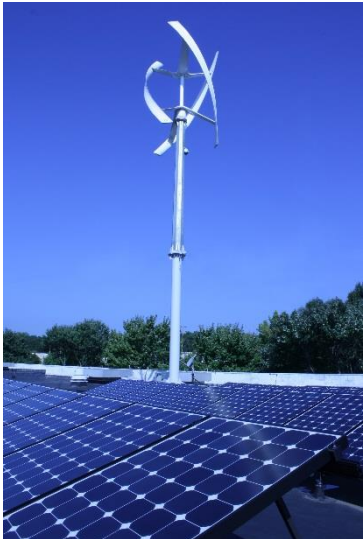
University Research Park's Environmental Way rooftop
